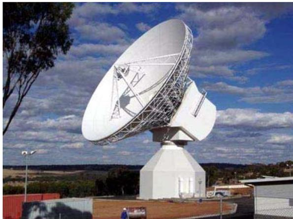
Figure 51: ESA New Norcia (Australia) 35 m deep space antenna.
