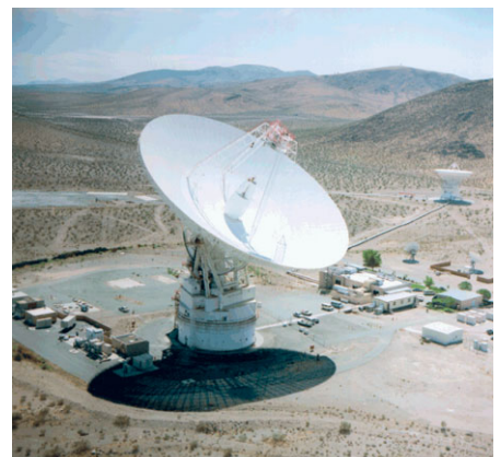
Fig. 16. NASA's 70 m (foreground) and 34 m (background) deep space antennas at the Goldstone complex in the Mojave desert. (NASA)
