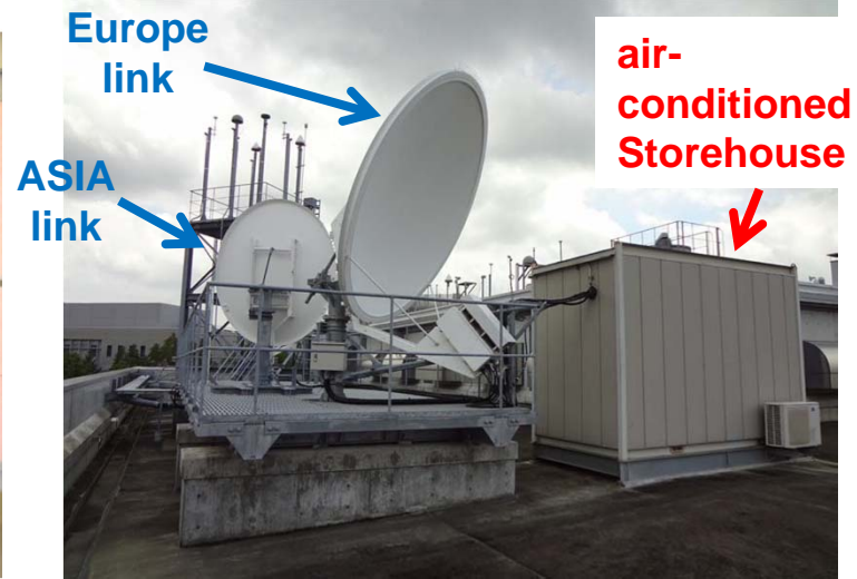
Earth station configuration
